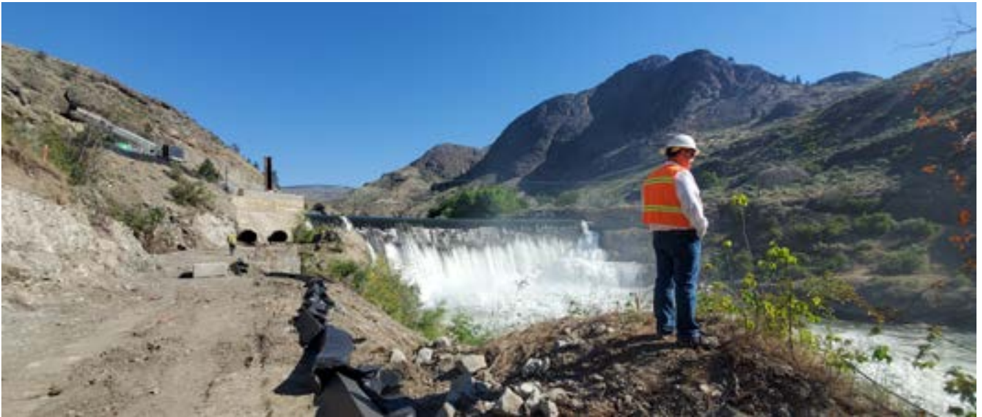
Okanogan PUD General Manager Steve Taylor at Enloe Dam.
