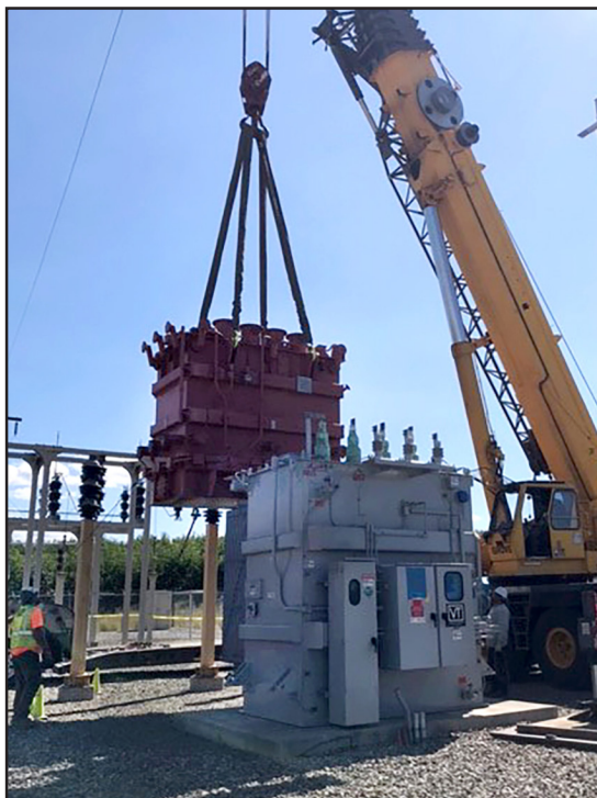
Left: The old power transformer (red) is hauled away as a new one is installed in the Omak substation.
