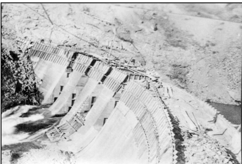
Enloe Dam while under construction, c. 1919-1920.
